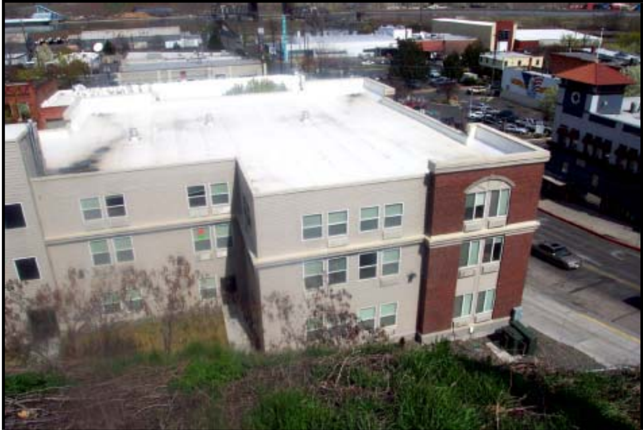
View north of the new building from the top of the steep hill to the south.
