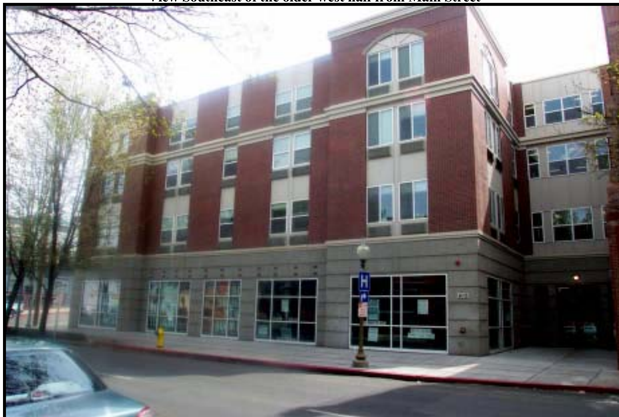
View southeast of new 4-Story building from Main Street
