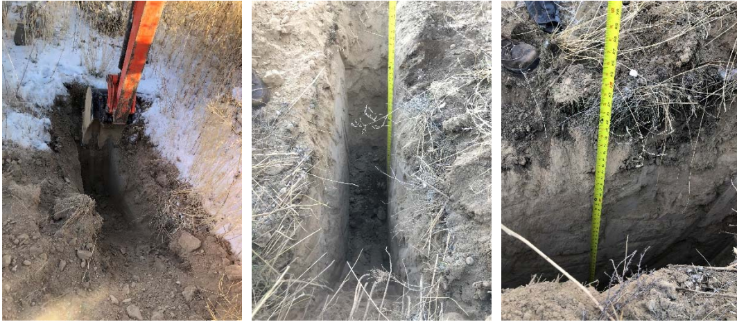
Figure 3. Test pits for soil sampling
