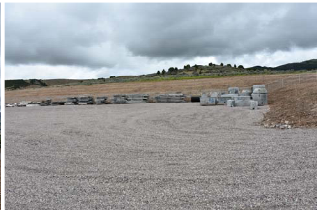
(f) Gravel pad for staging area
