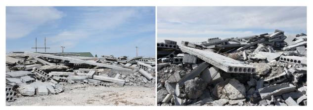
Figure 5. Precast concrete waste pile at Teton Prestress Concrete in Idaho Falls
