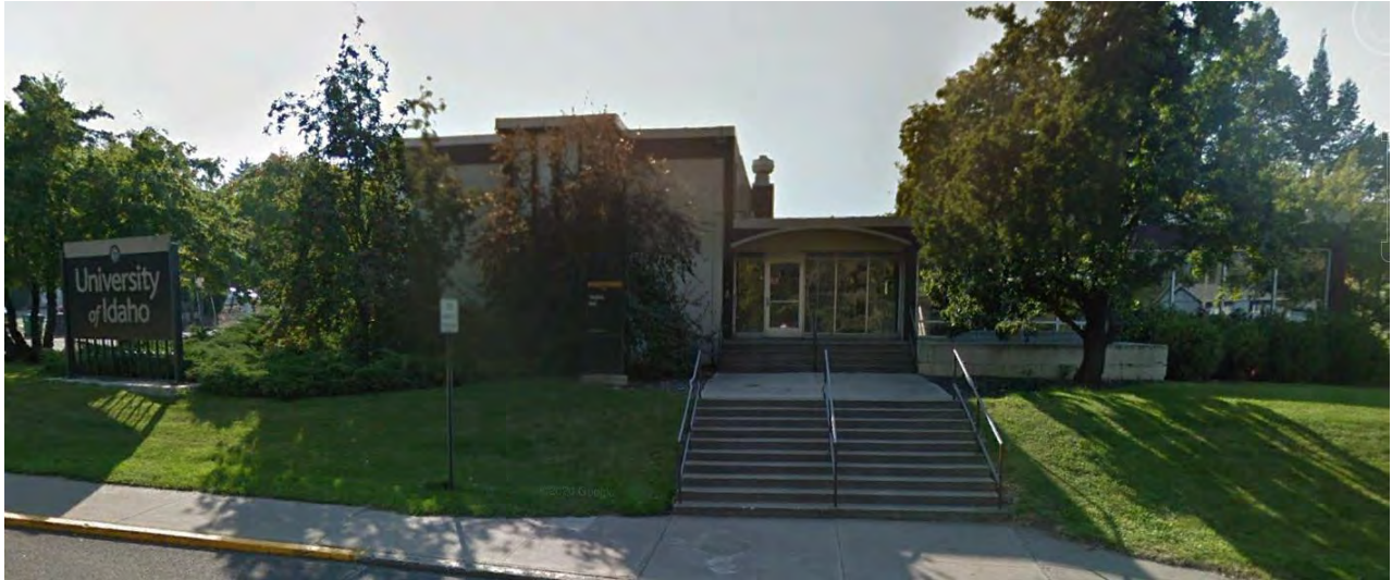
Existing Condition, Targhee Hall:
