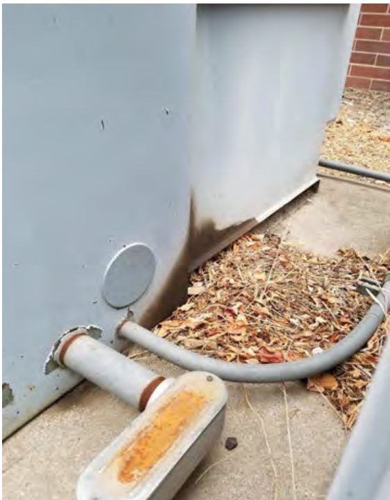
Figure 1. Example of oil leaking from transformer.
