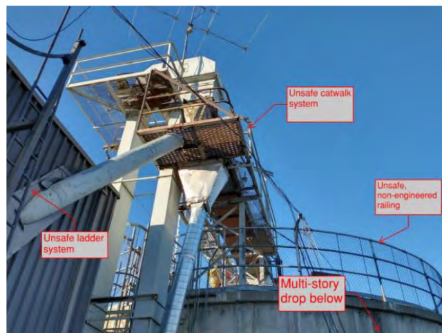
Figure 1. Unsafe ladder systems to service boiler exhaust stack and roof.
