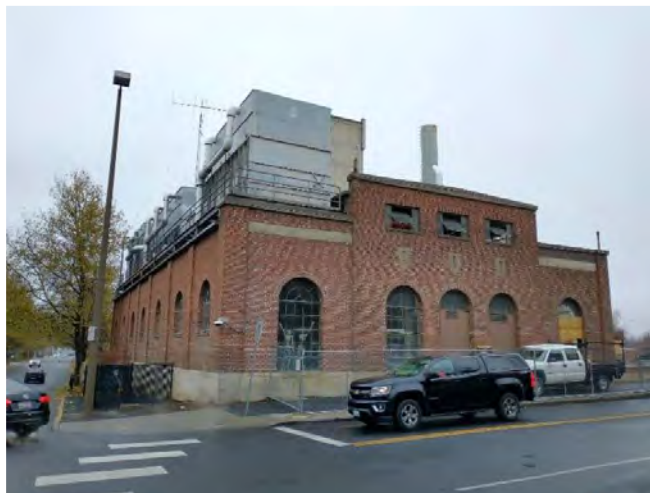
Figure 3. Brickwork at Energy Plant.
