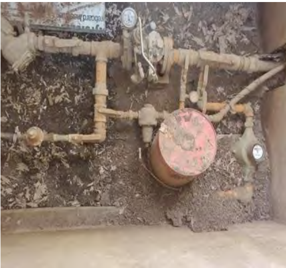
Figure 1. Interior vault at shed.
