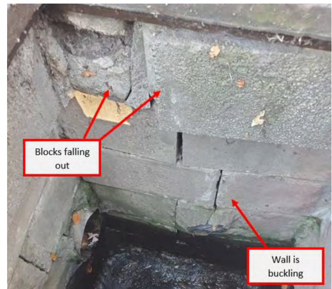
Figure 4. Catch basin at South Hill Apartments.
