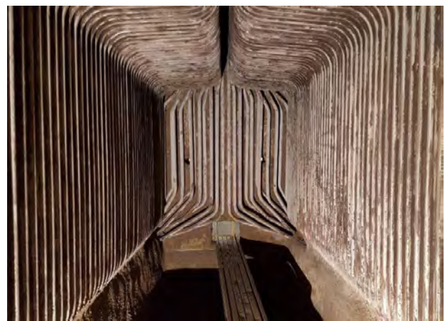
Figure 3. Condition of boiler tubes unknown.
