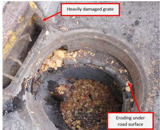
Figure 2. Catch basin on Rayburn.
