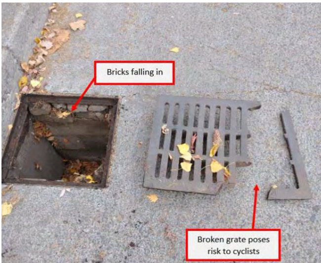
Figure 1. Catch basin on Campus Drive.
