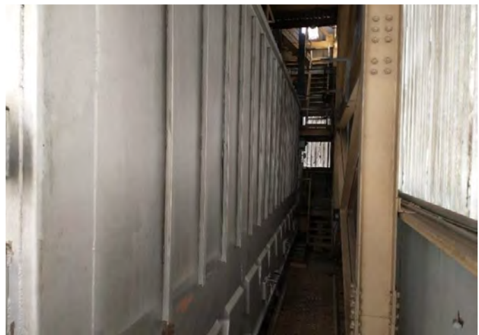
Figure 2. Non-insulated exterior walls.
