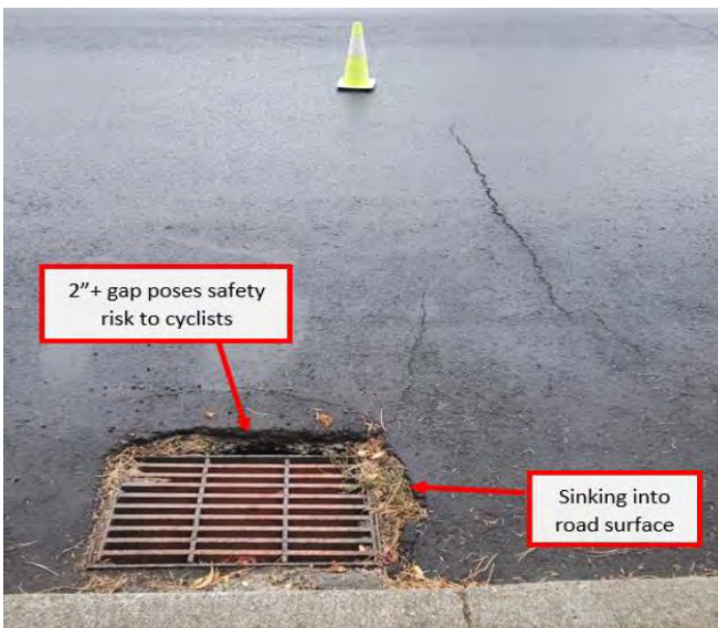
Figure 3. Catch basin on Perimeter Drive.
