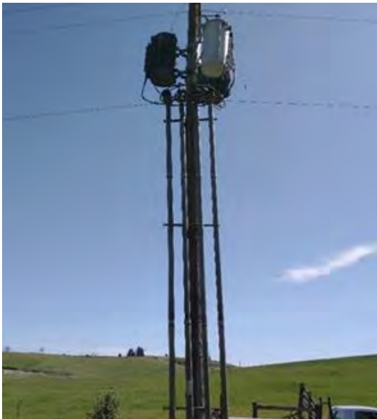
Figure 1. Aging poles, cross bars and mount transformers that pose failure risks.
