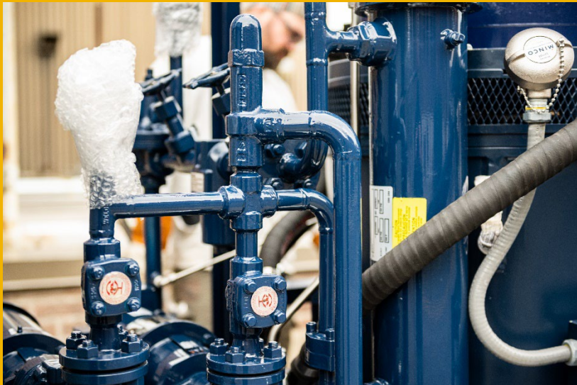
Steam plant microturbine installation
