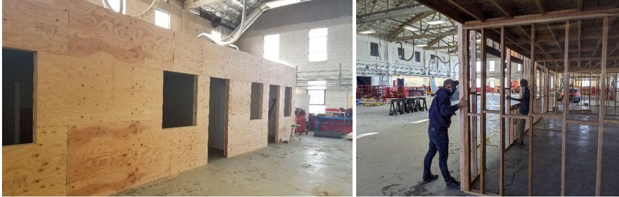
Figure 5. Construction of Mock-City Block in the indoor DRC
