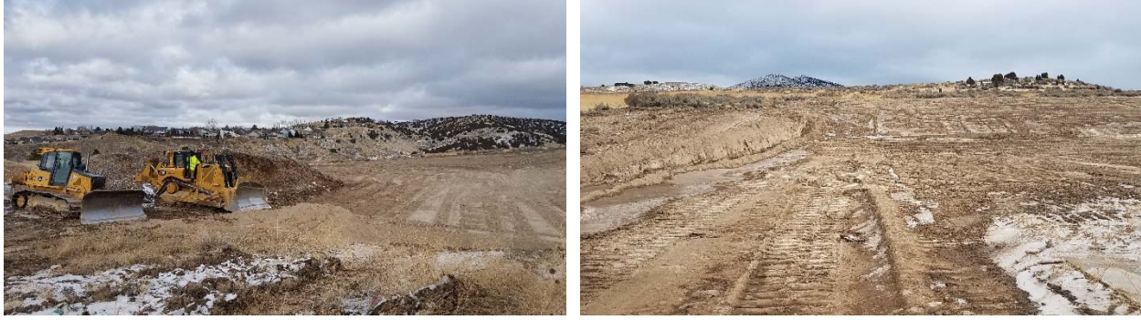
Figure 9. Ground breaking on December 30, 2019
