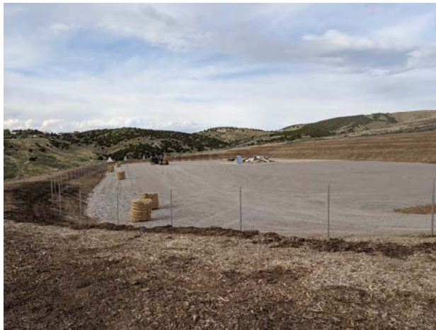
(a) Perimeter fence under construction
