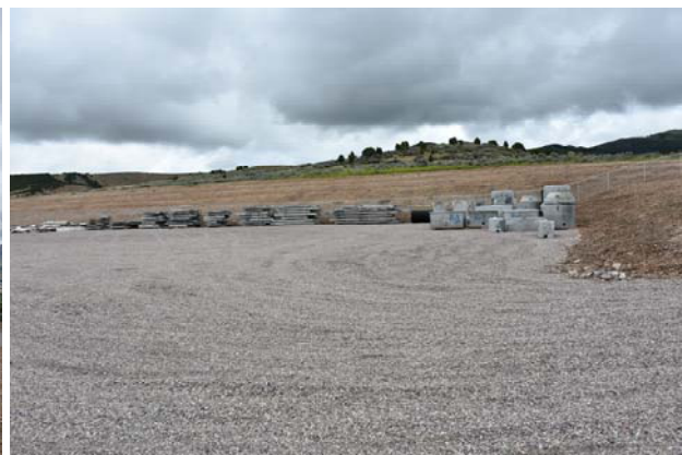
(f) Gravel pad for staging area
