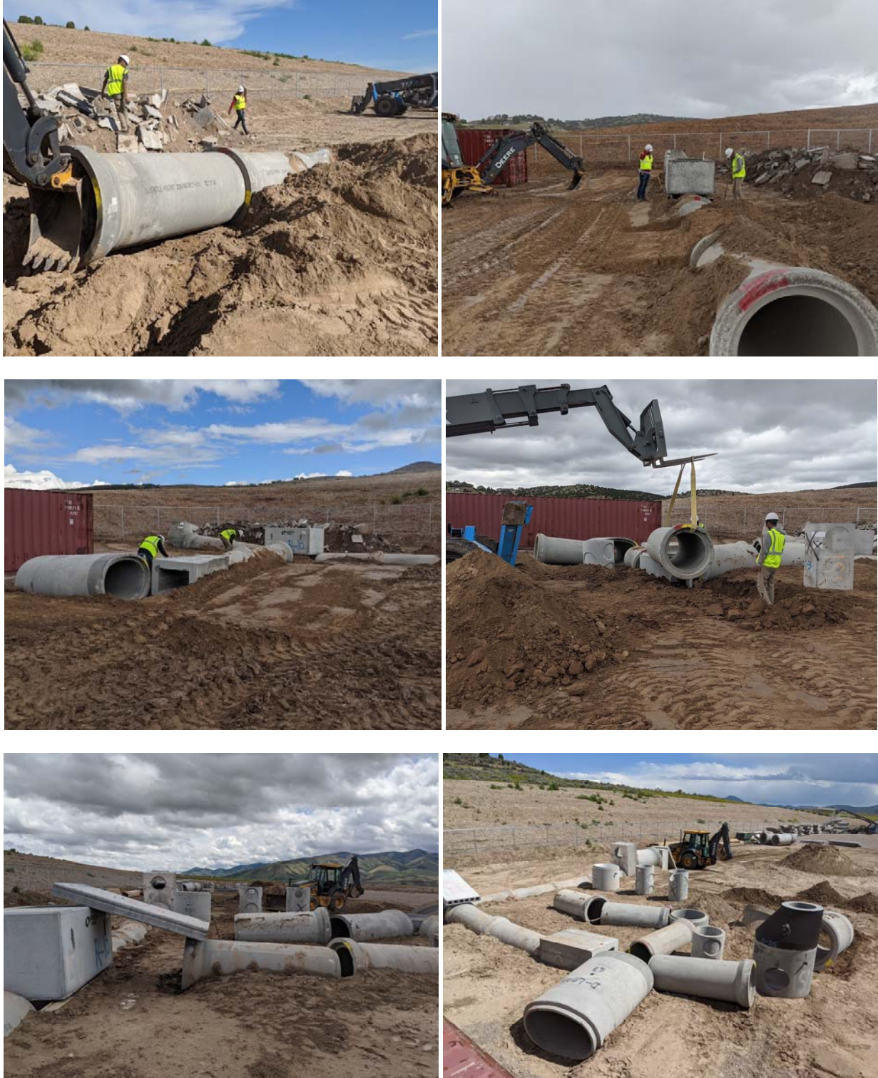
Figure 12. Photos from construction of subterranean lane
