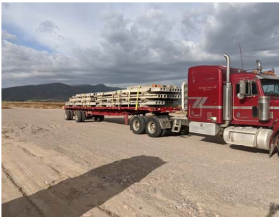
(c) Transfer of precast concrete sections
