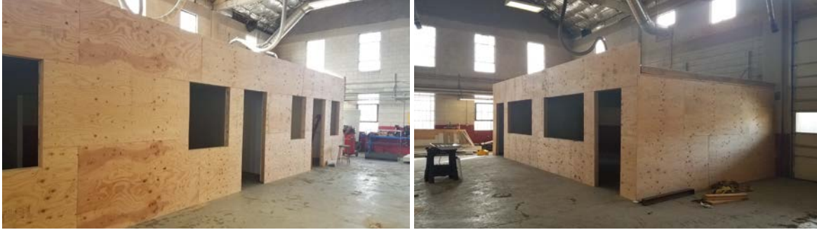
Figure 5. Construction is underway for Mock-City Block in the indoor DRC
