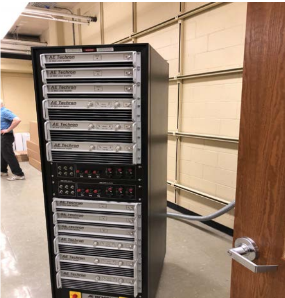
Figure 3: Amplifiers moved and installed in the new space.
