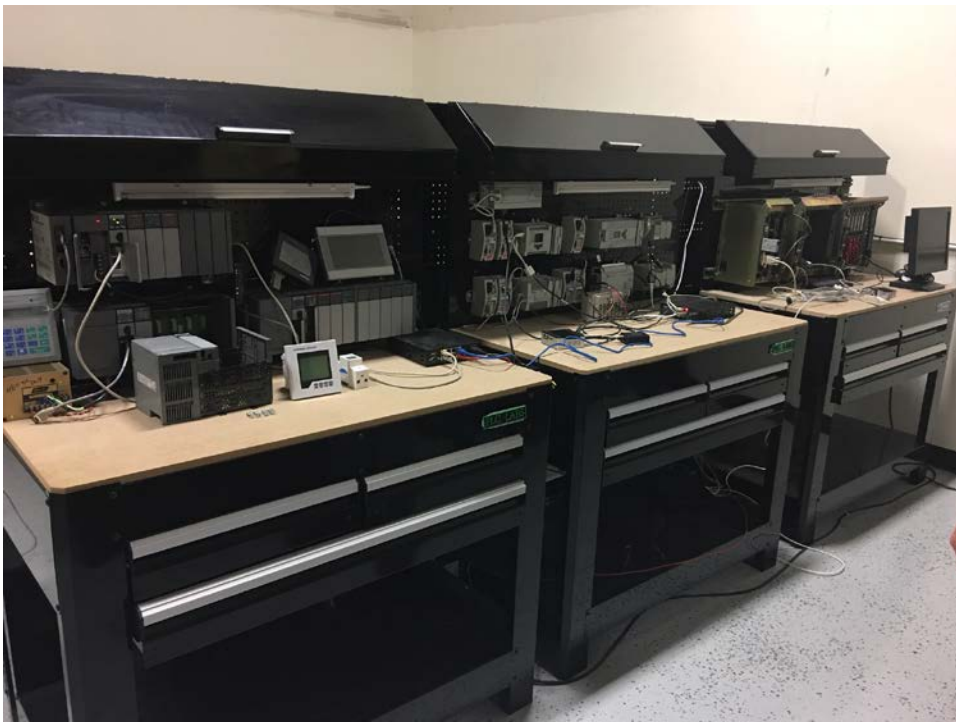
Figure 13: Kobalt workbench with HMI and PLC for Asset.
