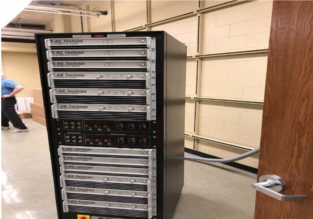
Figure 2: Amplifiers moved and installed in the new PowerLab space.
