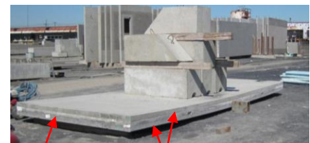
Foam Concrete Wythes Fig. 3. Bending Test of Insulated Precast Concrete Sandwich Panel
