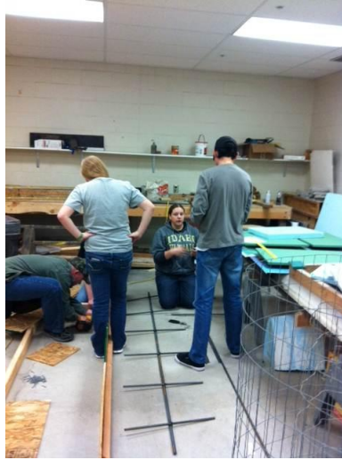
b: Rebar Assembling
