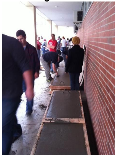
g: Constructed Panels
