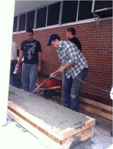
e: Concrete Vibrating
