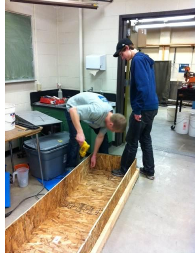
c: Formwork Construction
