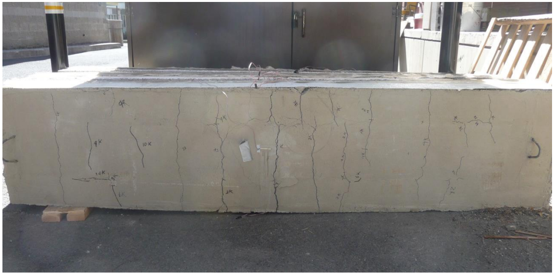
Figure 5: Bending Failure Crack Pattern
