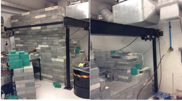
Figure 6 - Pictures of shielding around the production target area. The concrete bricks provide radiation shielding and the black iron is part of a rolling door and framing system
